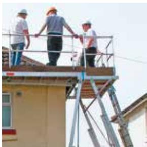
**Corner Kit:** Allows access to large box-end gutters or can provide a continuous working platform around corners.
