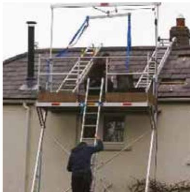
Solar Platform has been specifically designed to allow safe access up to roof level for solar installation, repair and maintenance. The Solar Platform is a 2m wide platform on adjustable legs with a rolling window bar, strap operated legs and a purpose designed hoist for lifting Solar Panels to roof level.
