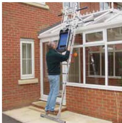
The Easi-Dec Conservatory Roof Access System is a specifically designed two piece system for accessing conservatory roofs, or any glazed roof, for cleaning and maintenance purposes.
