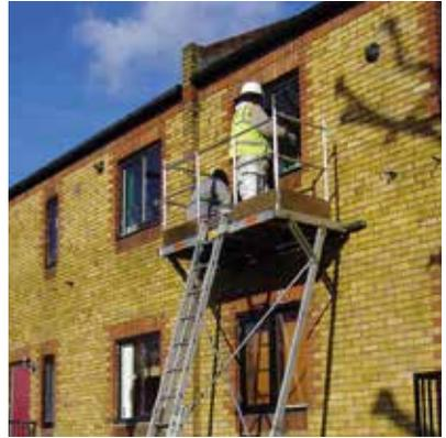
The original Easi-Dec platform provides safe, rapid access to roofline level, whilst spanning building obstructions such as porches and windows.
