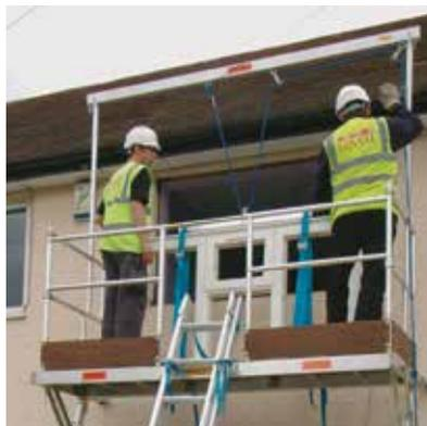
Window-Dec is a purpose designed platform which incorporates a lifting mechanism for window replacement. The fully protected work platform has an opening in the base to allow windows to be lifted through, safely and securely.
