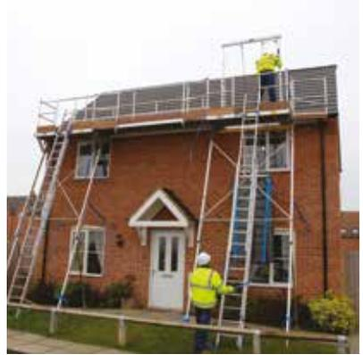
The Solar Access System provides a safe working platform combined with certified edge protection at roof level. The system comprises one Solar Platform, one Easi-Dec platform and a Catwalk which provides either an 8m or 10m long working area. Additional Decs and Catwalks can be added to provide a limitless modular system.
