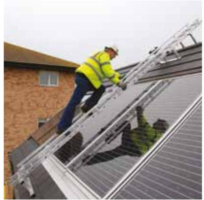
The Solar Ladder offers a safe, practical way of working when installing or maintaining solar panels. The bridging ladder provides 23cm clearance from the roof to the underside of the stile and up to 4.6m free span over the roof. The ladder is simply rolled up the roof on its soft rubber wheels and then flipped 90° into position on the roof. The ladder can also be easily traversed along the ridge with the use of special wheels fitted to the roof hooks.
