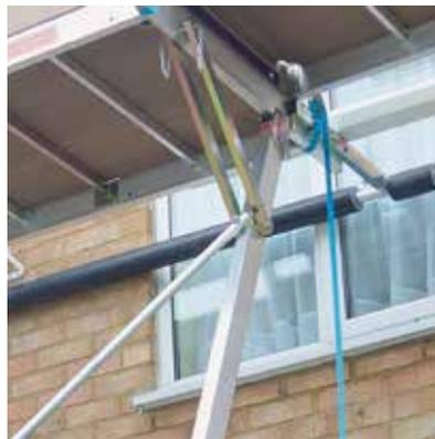
The Trimline System has been designed specifically for fascia, soffit or gutter replacement on standard sized homes.
