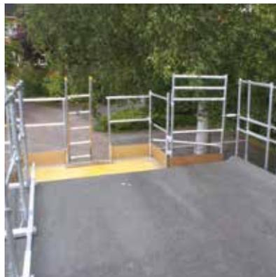
Our Low Level Roof Edge Protection system is designed to provide safe access and edge protection on low level roofs such as on a single garage roof or on a collection of flat roof units.
