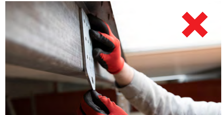
Fig. 1: Incorrect - bracket bends towards you
