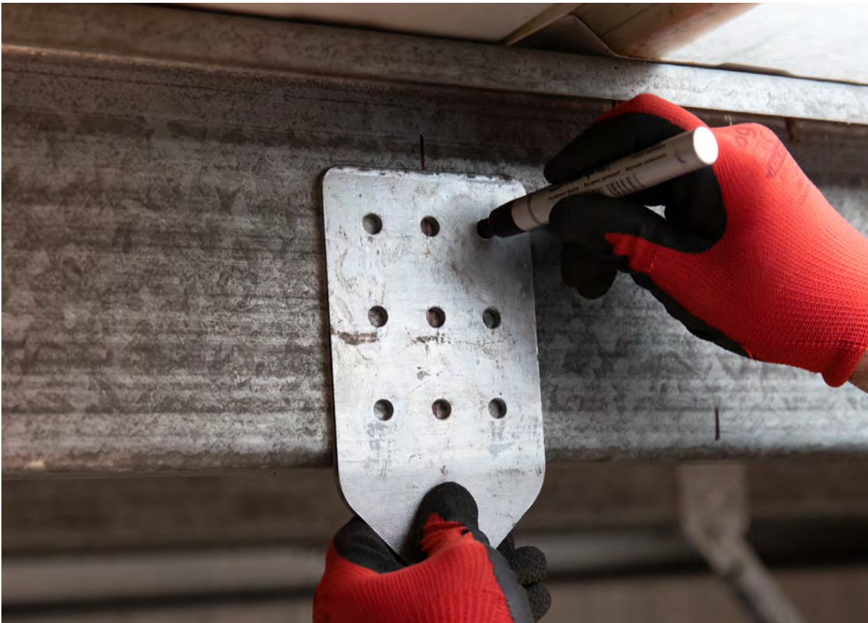
Fig. 1: Incorrect - bracket bends towards you
