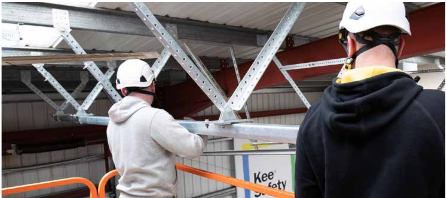
Two installers using an elevated platform secure the rail to the roof infrastructure.
