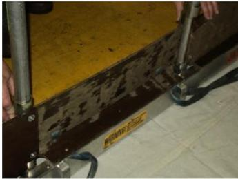
Raise the Toe Board across the ladder access point to complete the assembly.
