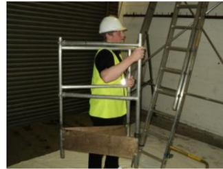
Position the Guardrail over your shoulder when climbing the Ladder maintaining three points of contact. **REMEMBER:** When installing the Guardrail to the right hand side of the Platform carry up on the right shoulder. These steps are repeated for the Left side.
