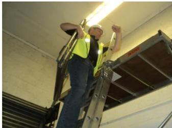
Feed one arm through the top rung of the Ladder. This provides a handhold when installing the Guardrail into position. **NOTE: This is why the Ladder needs to be extended above the platform by 3 feet (approximately 1 meter) to provide a handhold.**
