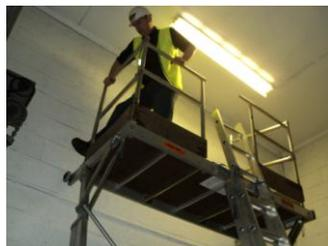
Climb onto the Platform and position the rear uprights into the rear locating sockets on the platform for both the Left and right hand Guardrail.
