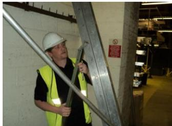
Remove top pin and attach the back Leg at about eye level.
