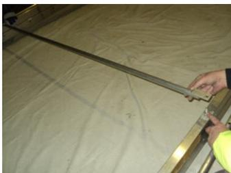
Slide the Horizontal Cross Brace holes over the retaining studs.
