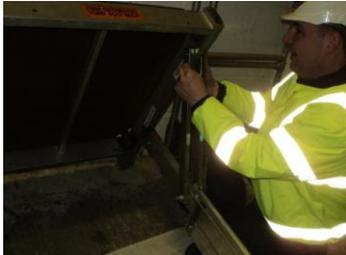
Rotate the Dec support struts and secure with the pins and 'R' Clips provided.
