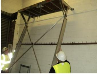
Lift the Easi-Dec up to waist height with bent legs and a straight back, first to waist height, then using your arms, place it against the wall and roll it up into position.
