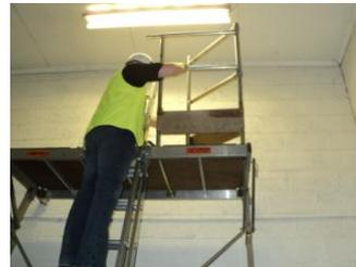
Insert the Right hand guardrail into the two front sockets and gently ease the back of the Guardrail open. **REMEMBER:** Always have your arm through the top rung of the Ladder when positioning the guardrails. Repeat these steps for the Left hand Guard rail.
