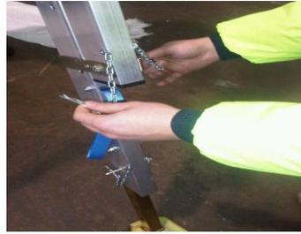
Adjust the height by removing the two Leg Pins and rolling the Easi-Dec up the wall to the desired height and replace both Leg pins remembering to also replace the safety 'R' Clips provided. After adjusting to height it will be necessary to re-level the Easi-Dec by moving the feet either away or towards the wall.
